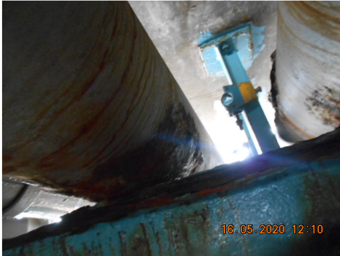
Corrosion on both of the 12" pipes
