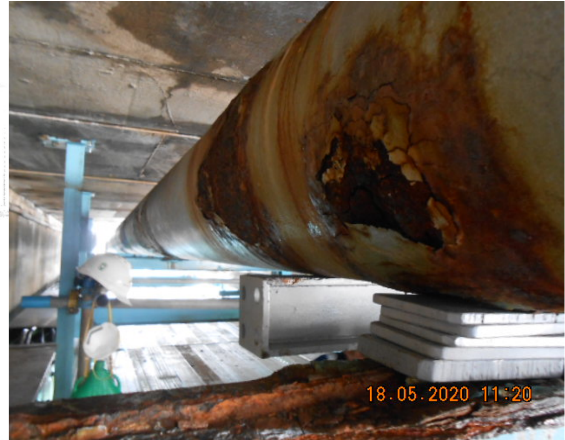
Both pipes required to be wrapped at 5m and 2.4m length
